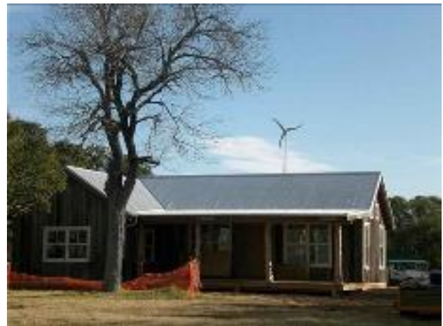
The ultra-efficient casita plans to meet its minimal electric needs with a 45-foot-tall 3.7 kW SkyStream wind turbine on a hill behind the house.
