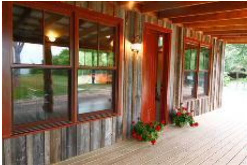
The front porch, built with salvaged cedar posts, extends the living space outdoors.
